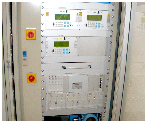
Figure 16 Quantity weight converter and measured value registration for the remote data inquiry of the reference meter section
