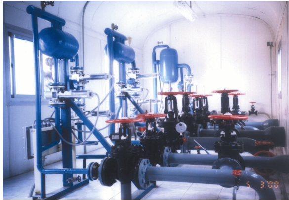
MFM 2000 series meters with and without Upstream Separation Device
