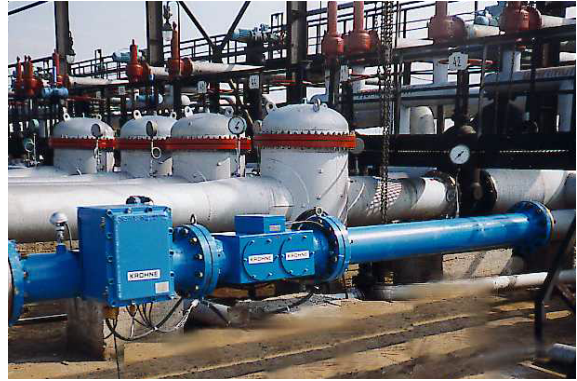
Figure 2: Application of an 8" Altosonic V on oil.
