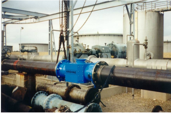
Figure 1: A calibration of a 16" Altosonic V on oil at SPSE in France.
