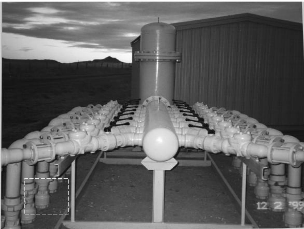
Figure 5a - Pod System V-Cone (16 units in same envelope as 7 orifice)
