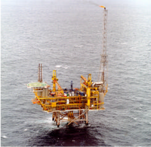
Fig. 21 - The Armada Platform
