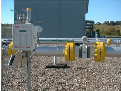
Fig. 18 - Picture of the installed 8”-meter in Kirchheilingen
