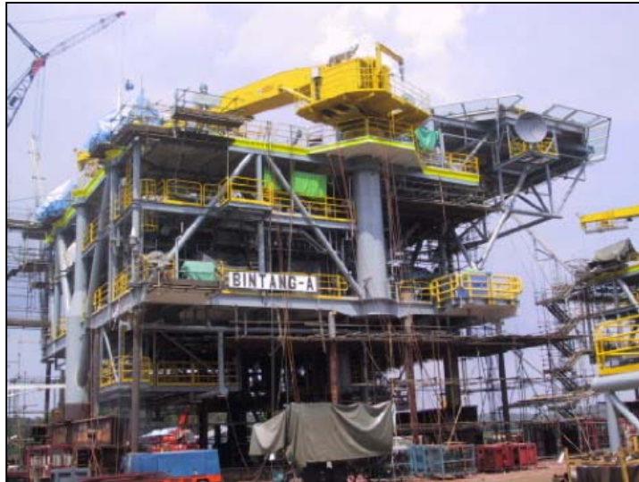
Figure 1. The Bintang-A platform under construction
