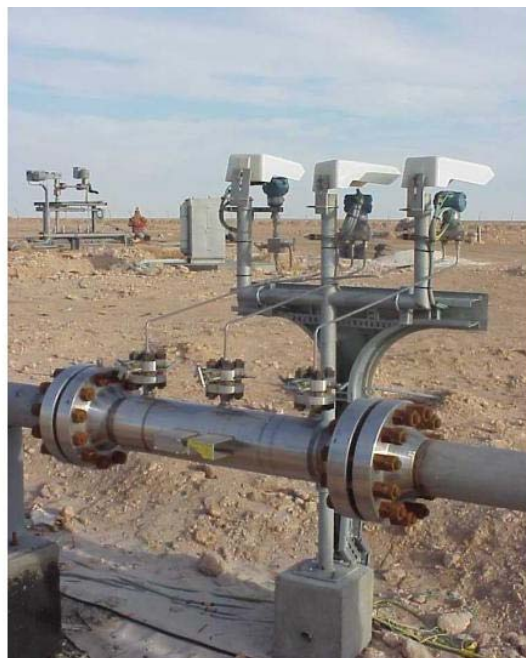
Figure 8, Wet gas Venturi.
