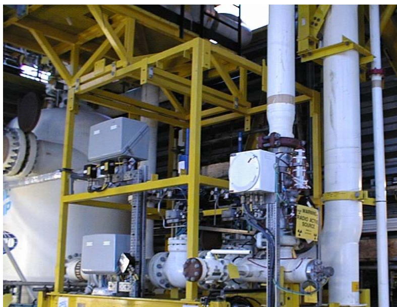
FIGURE 4:- PENGUIN METERING INSATLLATION – SEVERE SLUG SUPPRESSION DEVICE
