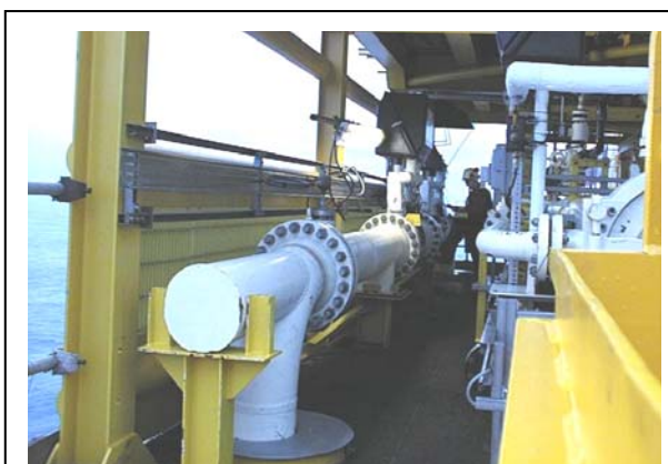
FIGURE 3:- PENGUIN METERING INSTALLATION – THE INSTALLED DS II METER
