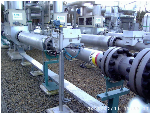
Figure 2 Meter section with vortex flowmeter prior to modification
