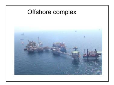
The water depth is shallow compared to European standards, typically 10 - 40 meters. The field is developed by small satellite platforms with 1 to 9 wellheads on each. Platforms are generally minimum facilities, with limited power and normally unmanned. The platforms are linked via a network of flowlines to a central processing facility.
