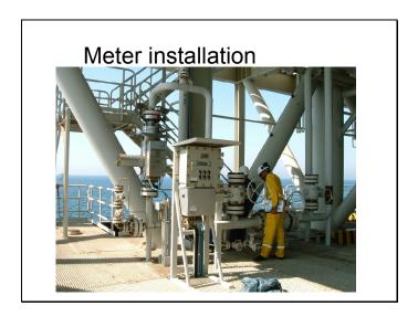
The picture shows one of the meters installed on a 9-well platform. The platform does not have safe area or control room. Therefore the flow computer is installed in a field enclosure close to the meter. The local display allows operators to directly read the flow rates, perform well tests and set up the meter in a simple way.
