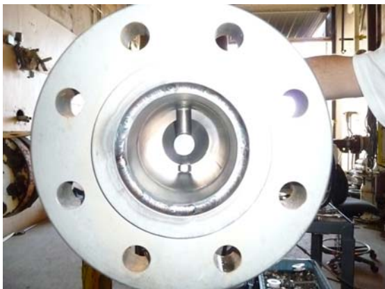
Fig 46. Trapped nut looking downstream
