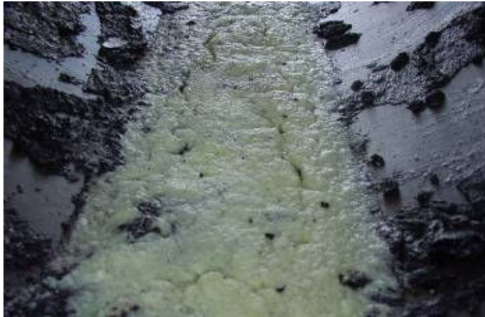
Figure 6, fouling as a flow on the bottom of the pipe.
