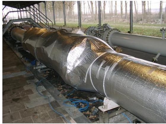
Figure 12 - Thermal lagging detail; Jan. 9 th 2009
