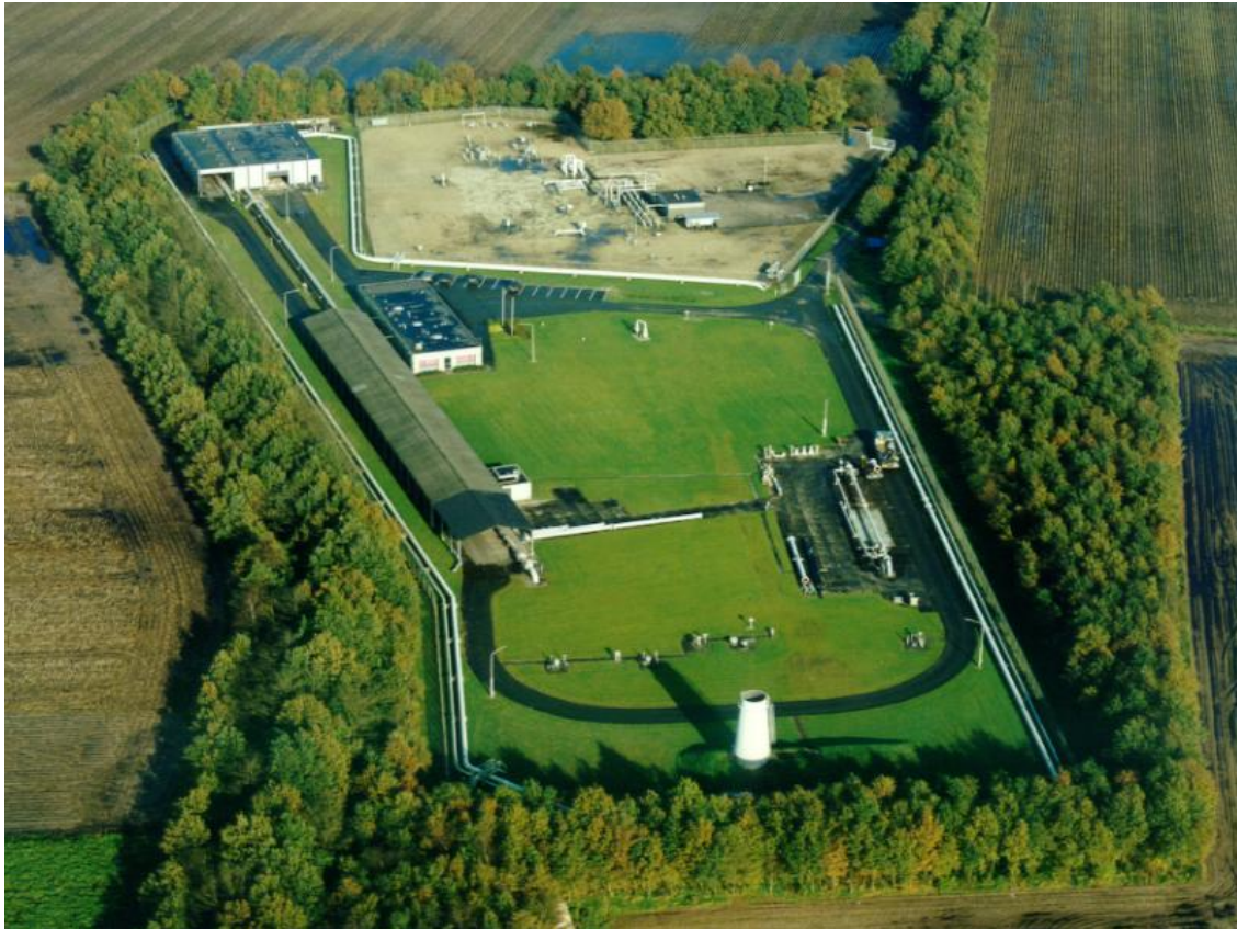
Figure 1 - Aerial overview of the Bernoulli laboratory in Westerbork, the Netherlands
