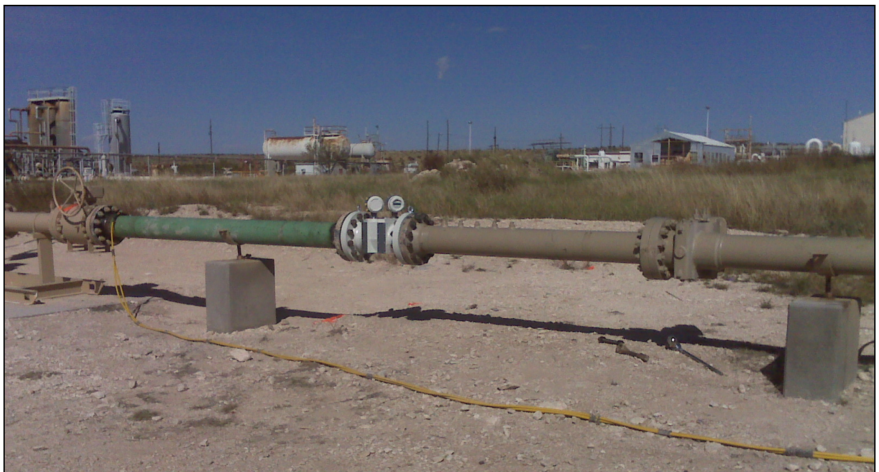
Figure 12: Test installation set up
