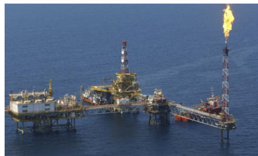
Fig. 1 – Gas flaring from an offshore oil and gas platform
