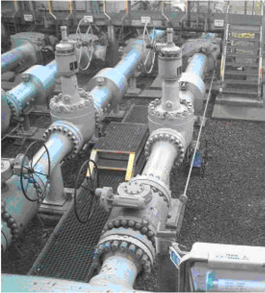
Fig.19 BP CATS upstream orifice run.
