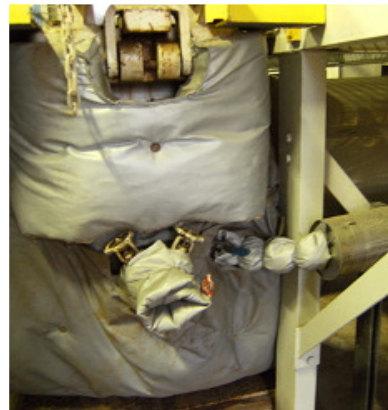
Fig.37a Corner Taps on CoP 36" orifice meter. Fig.37b Re-injection port downstream of plate.
