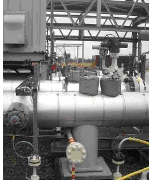
Fig.20 BP CATS downstream tap set up.
