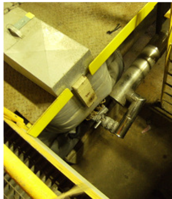
Fig.37a Corner Taps on CoP 36" orifice meter. Fig.37b Re-injection port downstream of plate.
