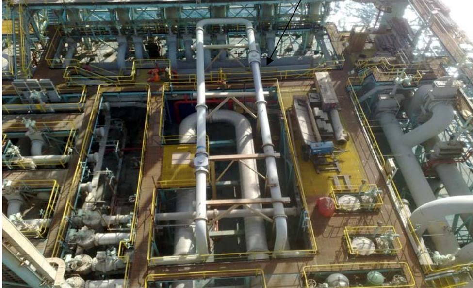
Fig. 6 U-Shape arrangement with three meters in series
