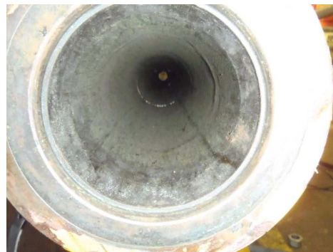
Figure 15:- Meter spool relatively clean
