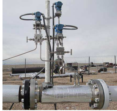
Fig 23. 8",sch 80, 0.75 \beta cone meter.
