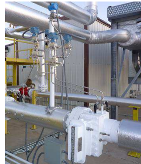
Fig 25. 8",sch 40, 0.69 \beta orifice meter.
