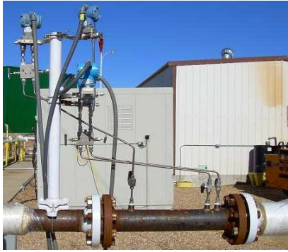
Fig 22. 4",sch 80, 0.63 \beta cone meter.
