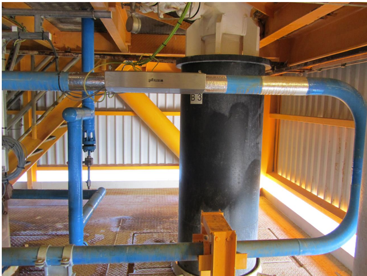
Figure 8 - Flag piping on K9-B; note transducer installation and damping material
