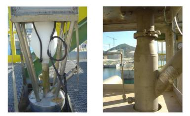
Figure 3 LNG sampling probes with effective (right) and less effective (left) insulation [Courtesy of Enagas]
