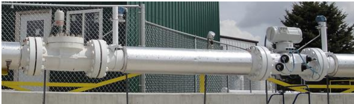
Fig 1. Gas Ultrasonic Check Meter Upstream of Primary Gas Turbine Meter.
