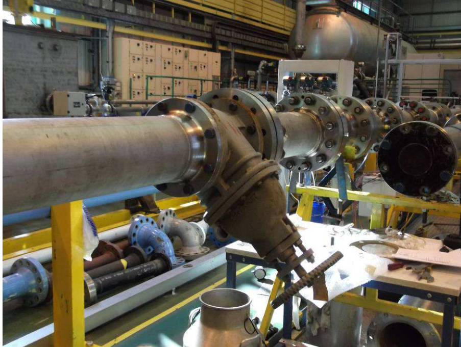
Figure 8 Simulation of a partially blocked flow conditioner (using a partly closed gate valve)
