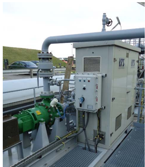
Figure 14: Field installation of e-Jetmixer
