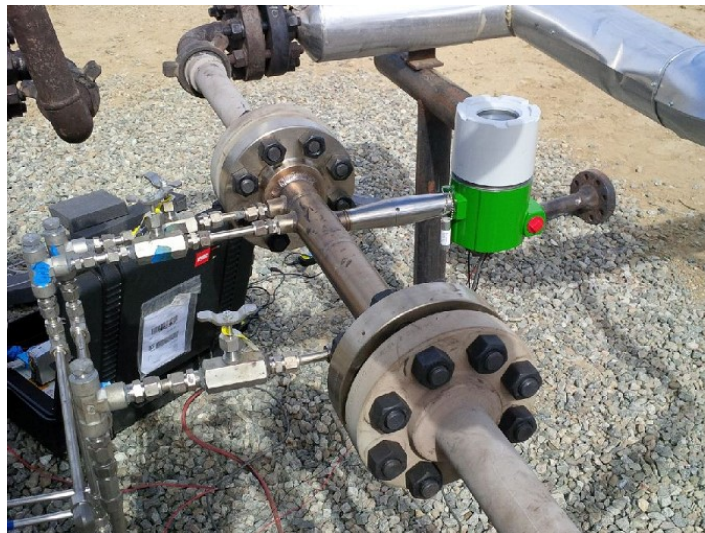
Fig 15. 2", 0.5 \beta VorCone Meter Saturated Steam Meter at the Injection Point.
