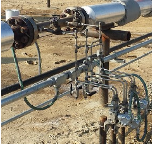
Figure 19. 4", 0.75 \beta VorCone Meter Installed At Steam Boiler Outlet.
