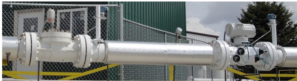
Fig 2. 8" Check Ultrasonic Meter Upstream of a Primary Turbine Meter.
