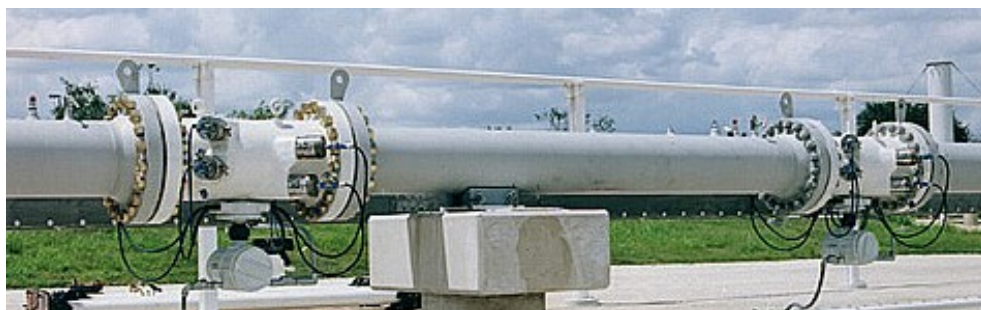
Figure 3. Check Metering with Two Ultrasonic Meters in Series
