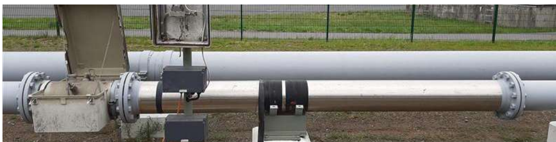
Figure 3a: Meter run before installation of the UFM.
