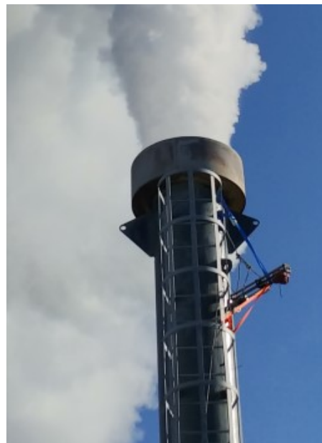
Fig 8. Separator Steam Outlet
