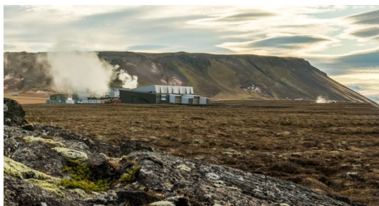
Fig 3. Theistareykir Power Station.
