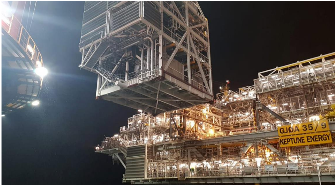
Figure 2: Lifting of the Nova production module onto Gjøa
