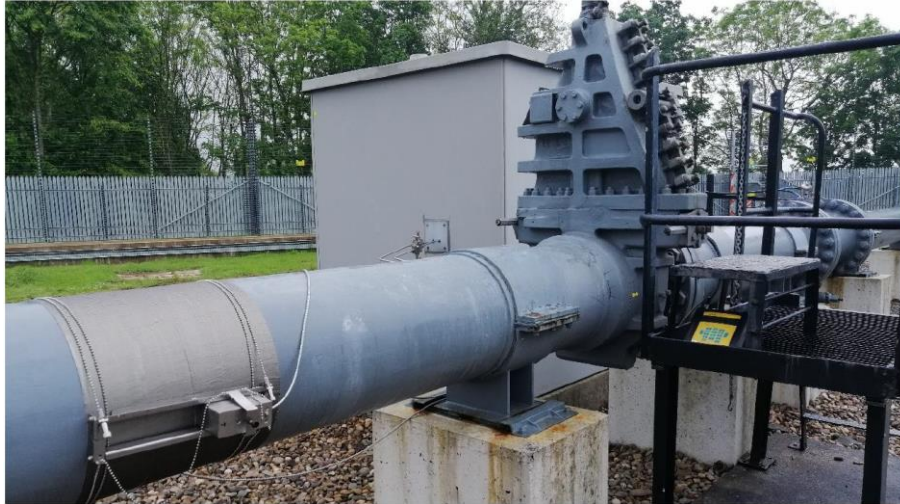
Figure 16 – Clamp-on USM Installation 5.2D Upstream to Orifice Plate Flow Meter
