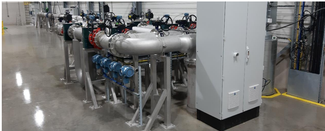
Picture 4 – WF2500 master meter sections
