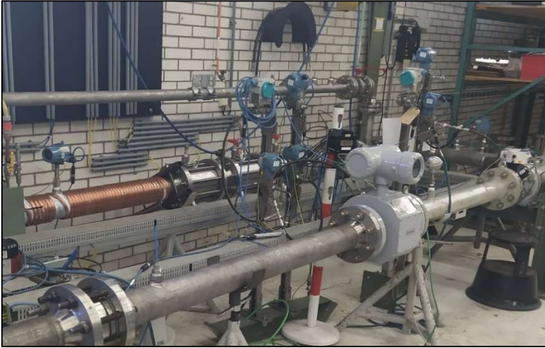
Fig. 5: A 4"/DN100 flowmeter at the DNV small hydrogen testloop.
